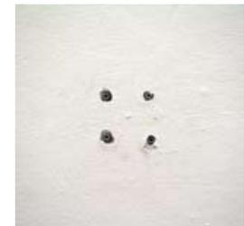
2) Drill four holes (6 millimeter in diameter) and insert wall plugs / screw anchors.
