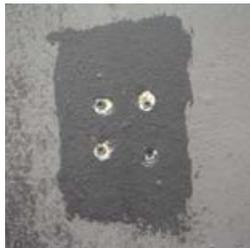
3) Apply one coat of shielding paint to area where the ground connection plate and grounding tape will be mounted. Allow ample time to dry.
