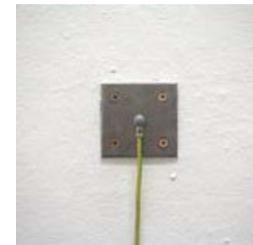
7) Connect cable to ground securely. E.g. use enclosed clip to connect cable to blank / bare heating pipe, or connect to grounding bar in outlet or fuse box.
